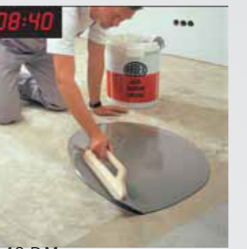
8:40 P.M. Use Hand Float to level the substrate quickly. 利用鏟板迅速整平基面
