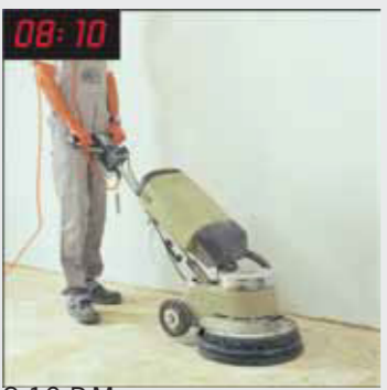
8:10 P.M. Removal of adhesives by grinder. 磨除殘膠
