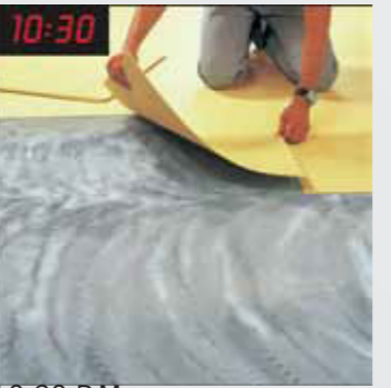
10:30 P.M. Install elastic floor covers. 逐步鋪貼彈性地材
