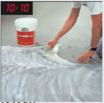
10:10 P.M. Apply adhesives for elastic floor covers. 開始刮膠鋪貼彈性地材
