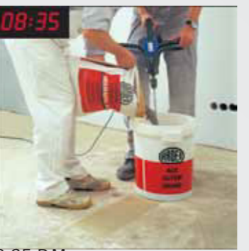
8:35 P.M. Mixing of ARDEX K55 Microtec Self-leveling Underlayment. 以機械攪拌方式拌合 ARDEX K55 超快乾鎖水自流平。
